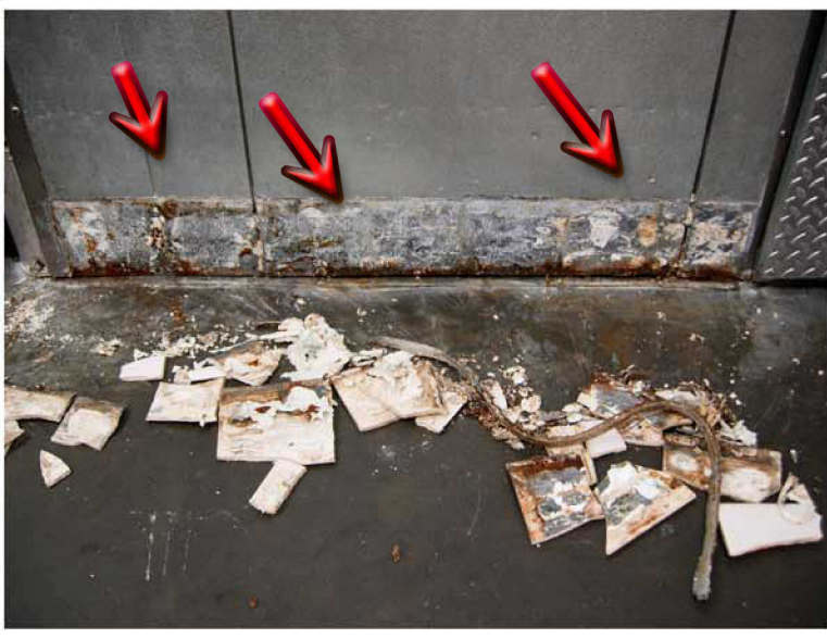
Bakery cove tile needs replacement and mold abated
