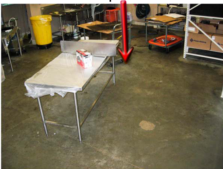
6"x6" non-slip tile never installed, employees slipping
