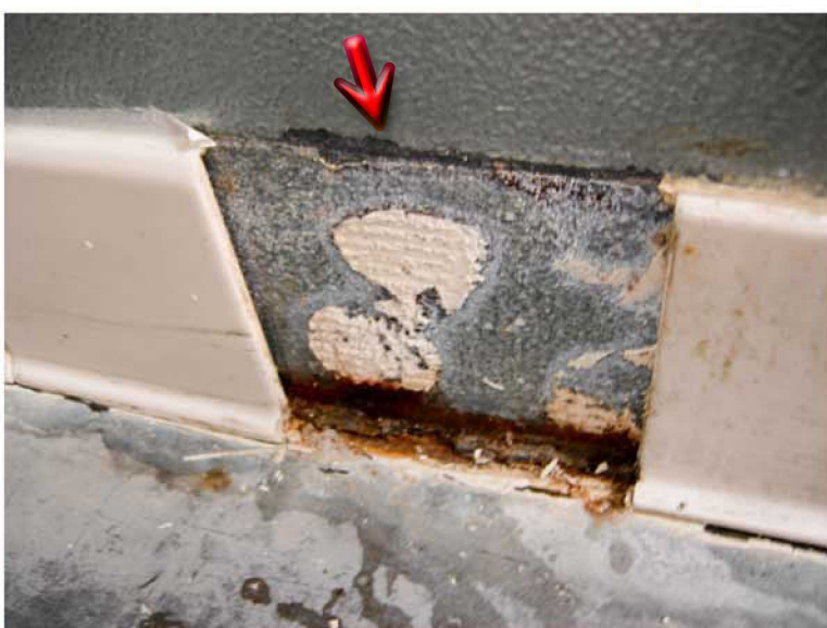
Bakery cove tile needs replacement and mold abated
