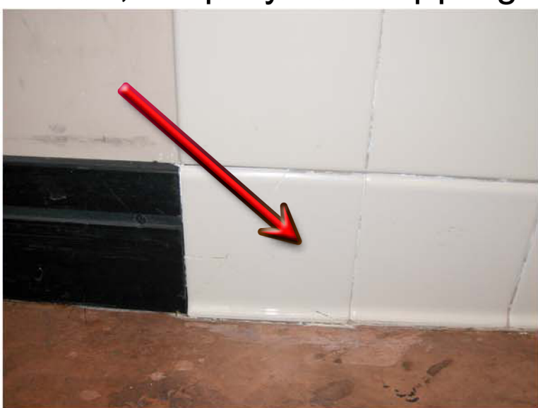
6"x6" non-slip tile never installed, employees slipping
