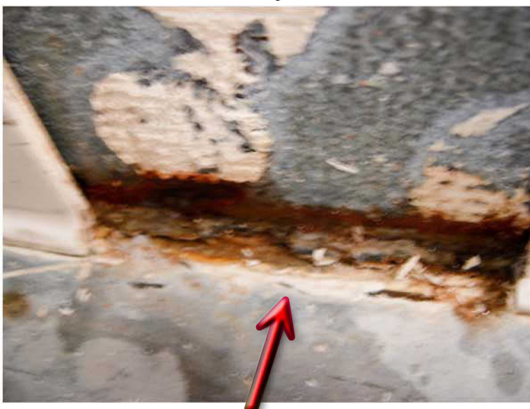
Bakery cove tile needs replacement and mold abated
