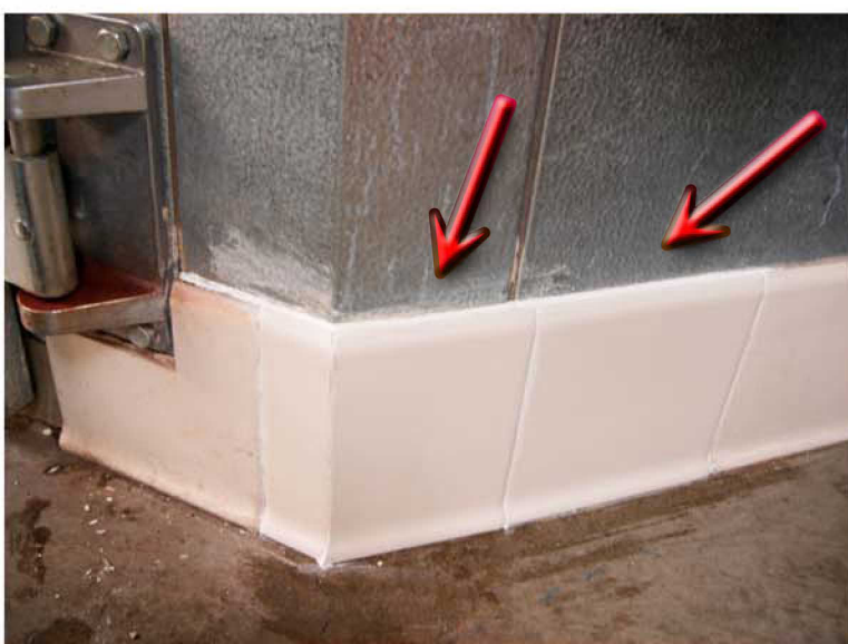
Bakery cove tile needs replacement and mold abated
