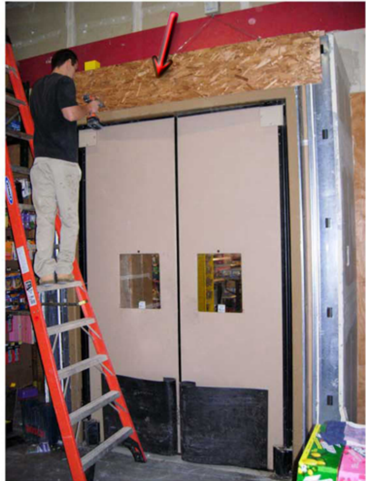
ADDING PLYWOOD FOR FUTURE STRENGTH
