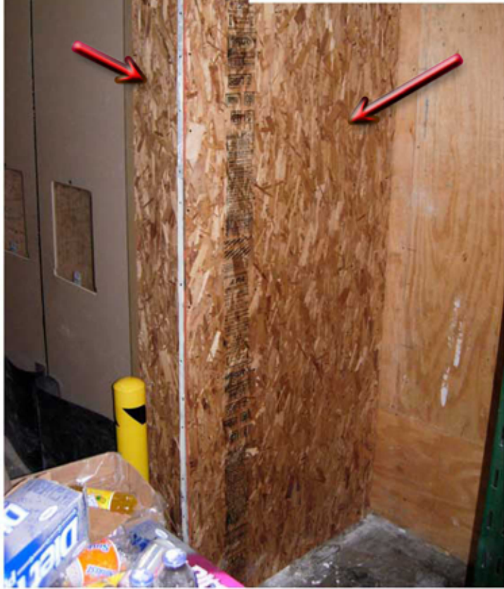
PLYWOOD ADDED TO SIDE WALL FOR PALLET PROTECTION
