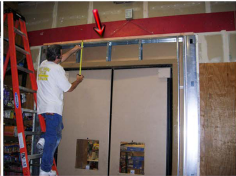
ADDING HEADER BOARD TO SUPPORT WALL
